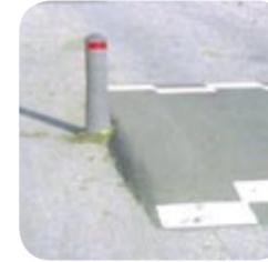
Bollards installed in conjunction with environmental obstacles to ensure that the cars cross the obstacle with both wheels whilst two-wheeled vehicles can pass without crossing the obstacle.
